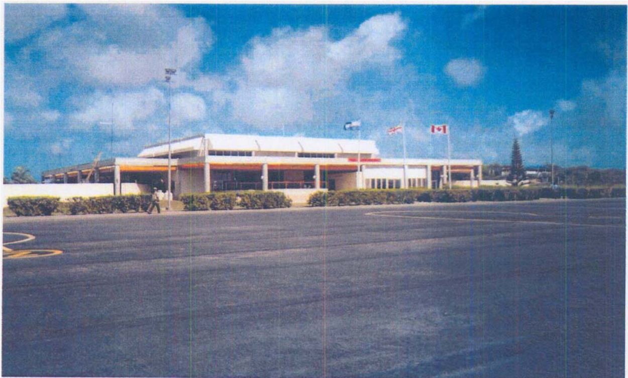
Photograph 4: Existing Terminal Building
