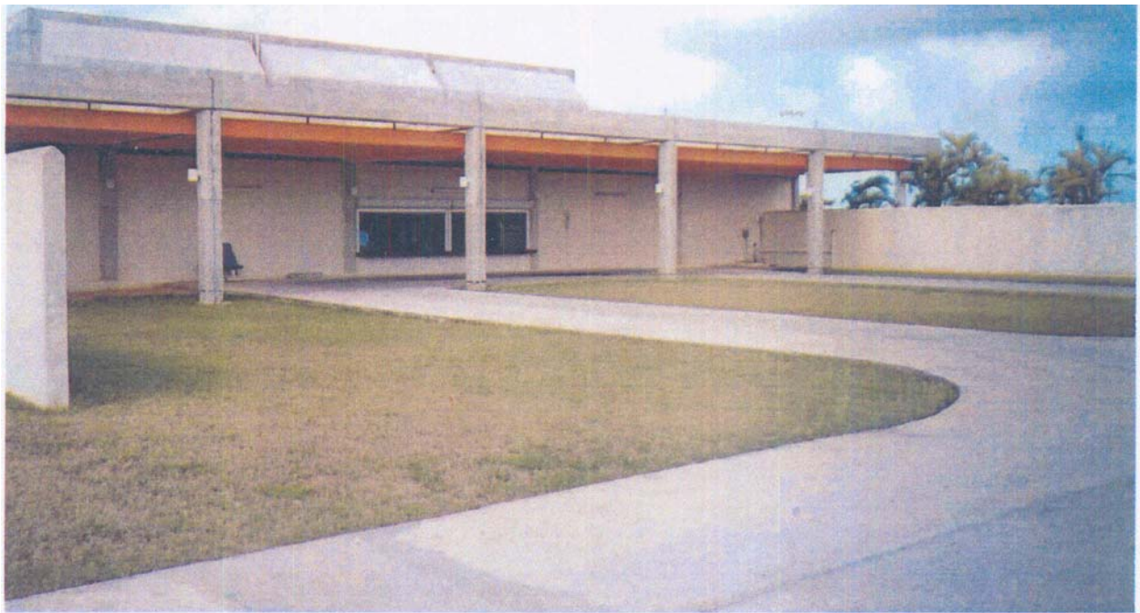
Photograph 11: Arrivals baggage unloading area
