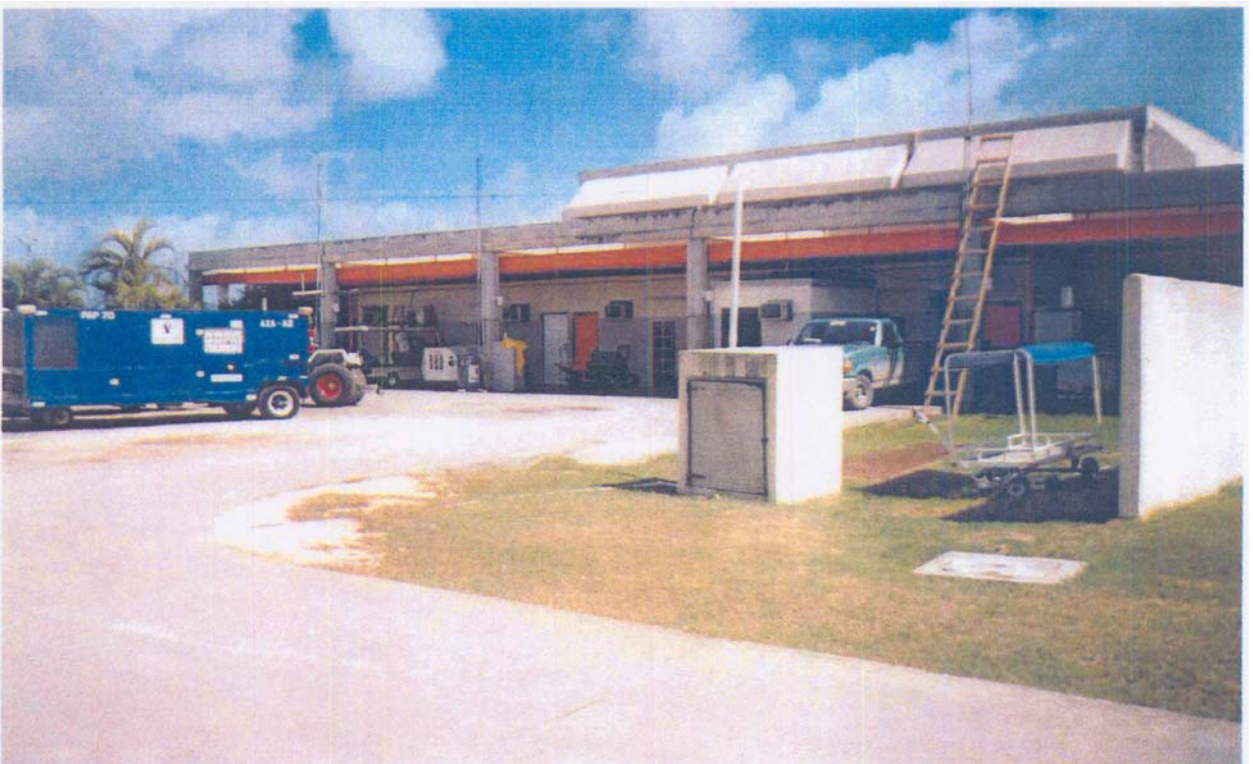
Photograph 6: Baggage handling area
