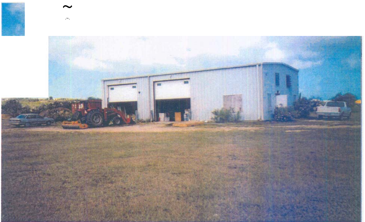
-Photograph 16: Airport Maintenance Facility
